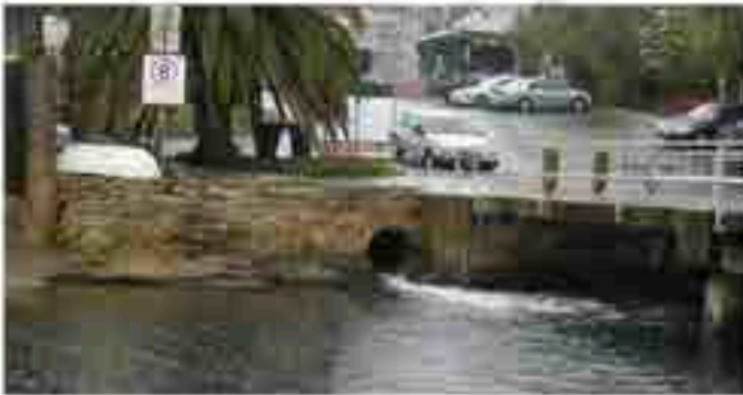
Storm water drain Photo: [unreadable]
