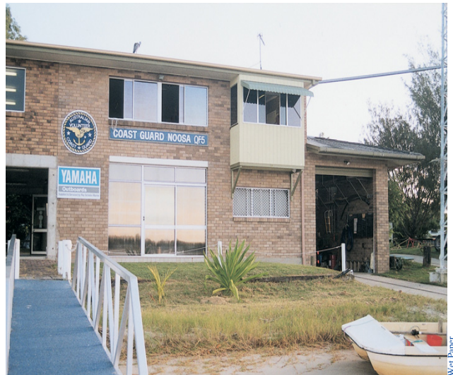
Figure 55.1 A limited coast station
