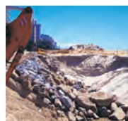
Boulder wall construction
